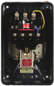
Interior View of MK1 DOL
