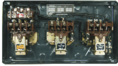
Interior View of MK2 FASD
